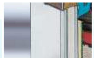
Corrosion protected by alocrom and epoxy painting.
