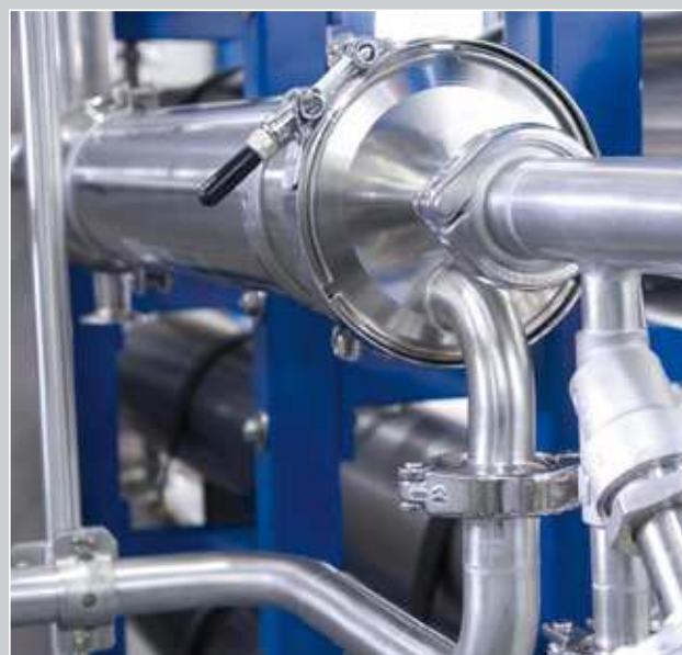
An optional membrane degassing stage removes high CO 2 concentrations.
