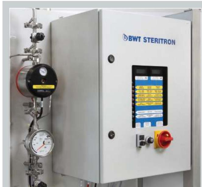
STERITRON ozone generation integrated into the LOOPO.
